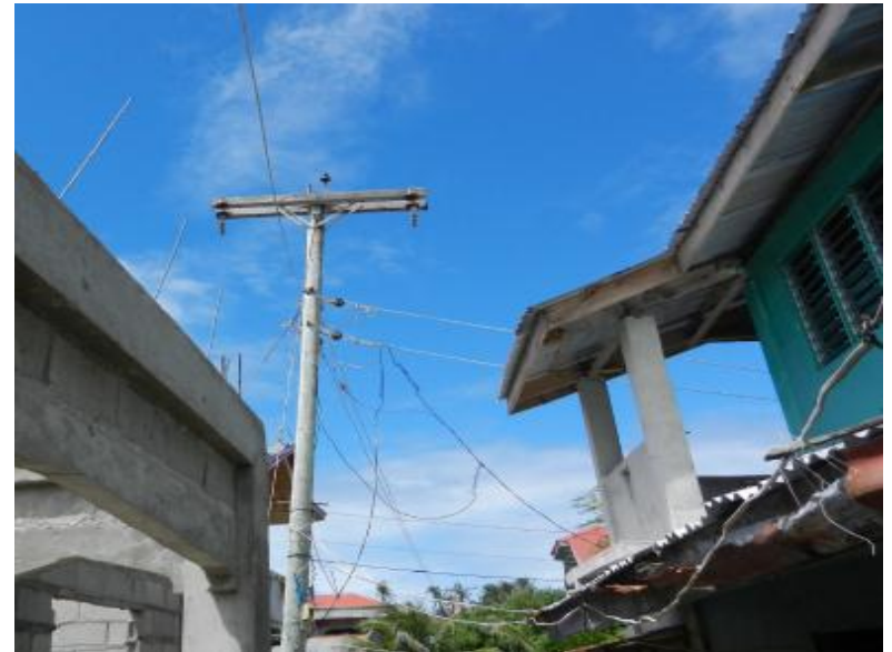
Wiring Network: making use of poles of old mini grid
