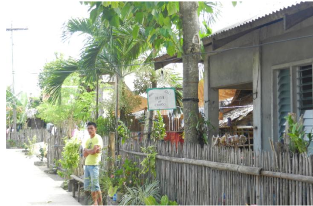
A typical wiring network around households
