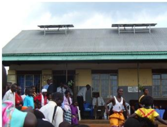
Health Centre with Solar Panel, Jinja District, Uganda
